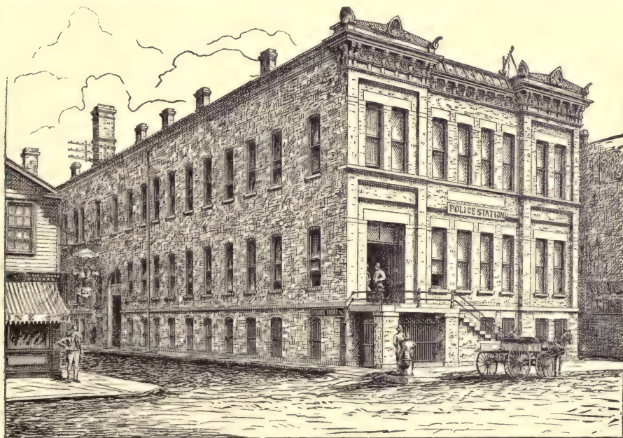
THE DESPLAINES STREET STATION.
