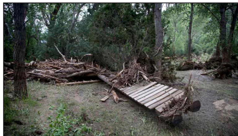
A bridge is displaced in middle Ponil canyon due to the flash flooding that occurred on Saturday, June 27. Cassidy Johnson/PhilNews
