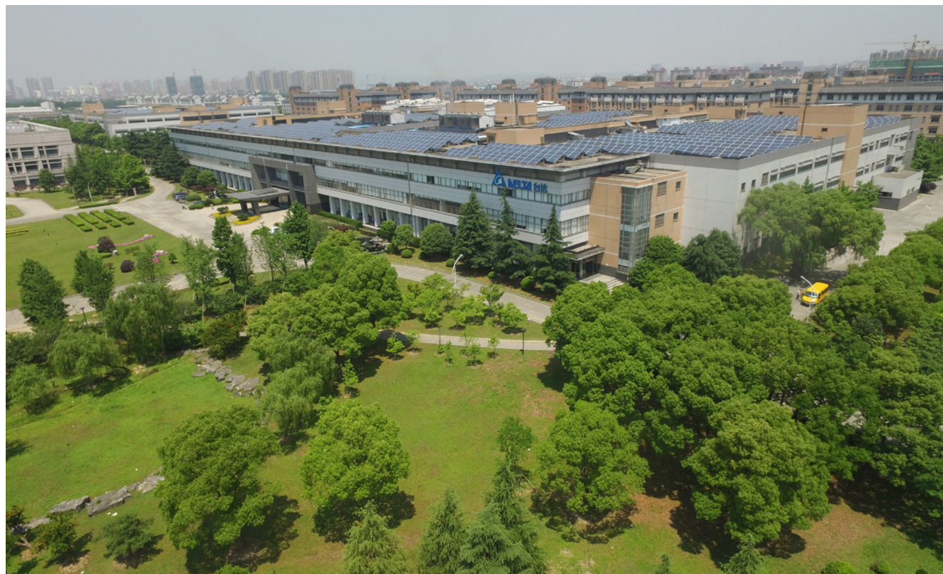
Delta's energy conservation plans in main production sites help achieve carbon reduction targets.
