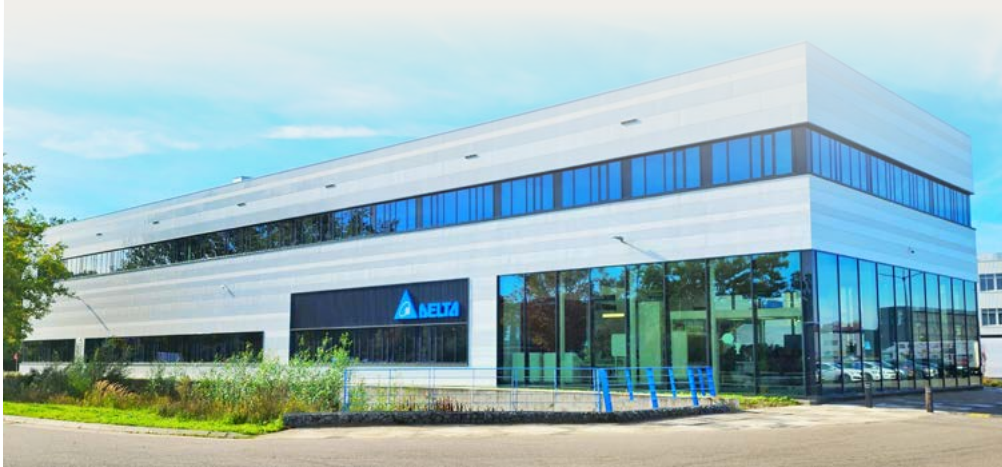
Delta's LEED Gold-certified green building at the Automotive Campus in Helmond, the Netherlands.
